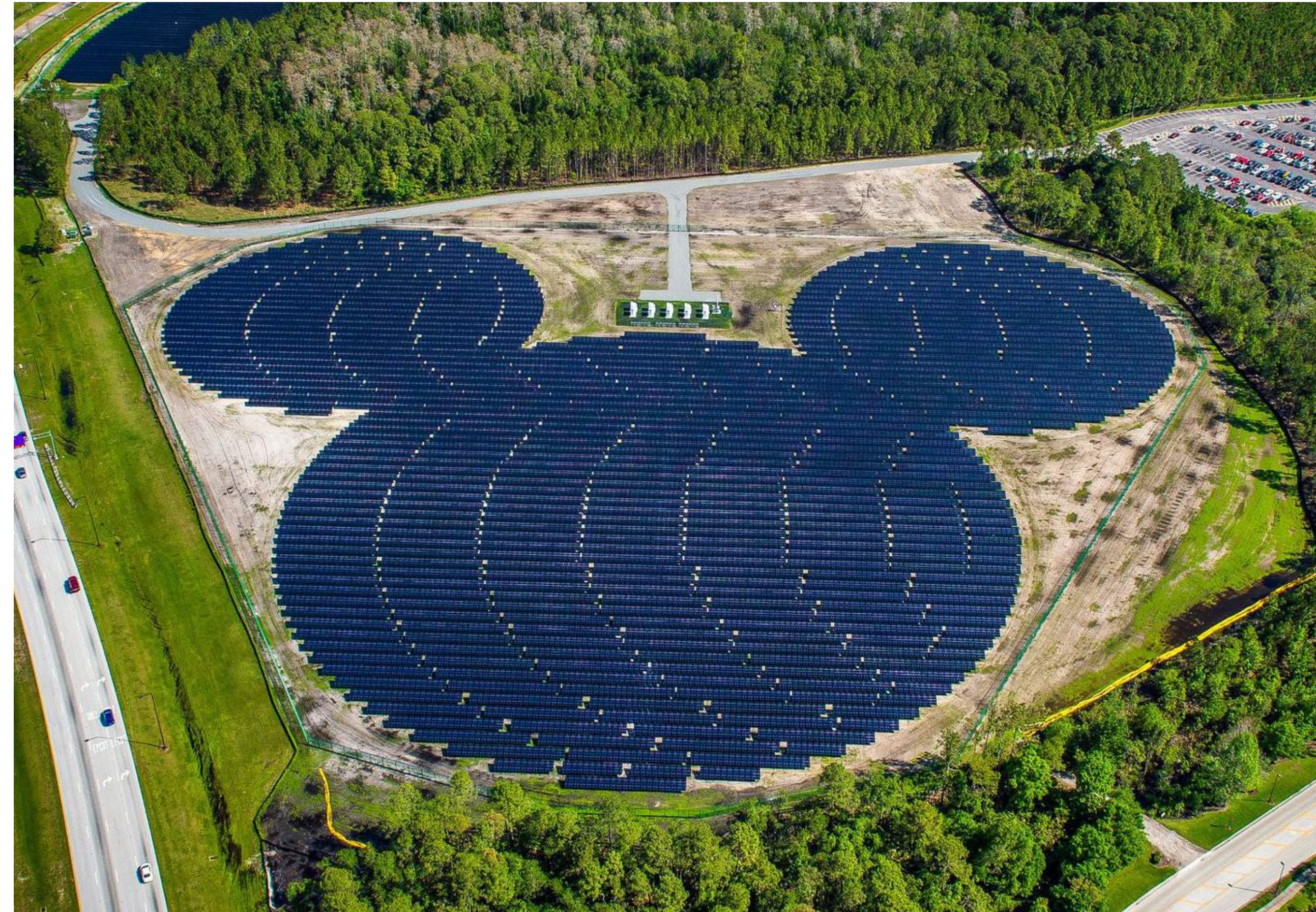
Solar array at Walt Disney World
